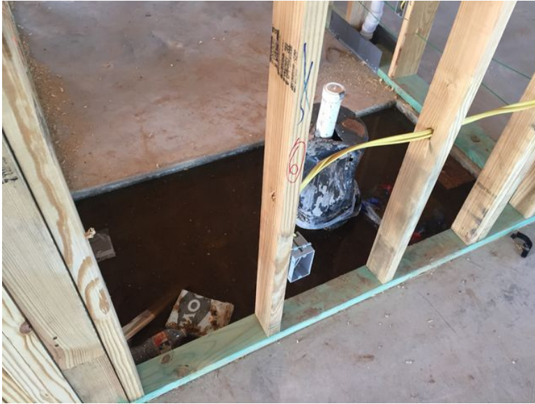
7. Drain lines are missing nail protector plates.
